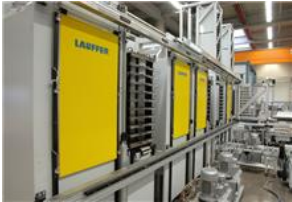
Installation and commissioning at a midwestern circuit board facility in May
